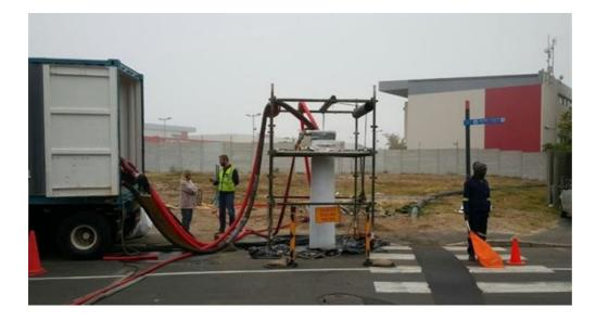
"A safe installation was implemented through excellent coordination and communication, with minimal impact and disruption to the public. The end result was a set of seven cost-effective, well-cured and rehabilitated close-fit lined sewer sections, with a total length of over 700m. The project was also achieved well within the programme schedule of the overall contract," Röhrs highlights.
