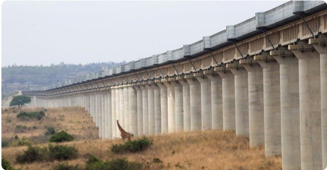
A giraffe walks near an elevated railway line that allows movement of animals below the Standard Gauge Railway (SGR) line linking Nairobi and Naivasha, inside the Nairobi National Park, in Nairobi, Kenya. Reuters
