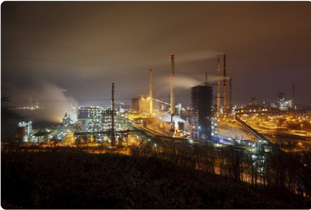
Power station in Accra. Source: Supplied
