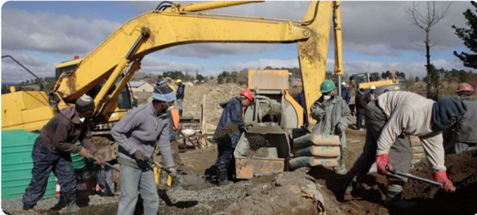
Construction of Maseru Maqalika Water Intake System in Lesotho. Image ©
