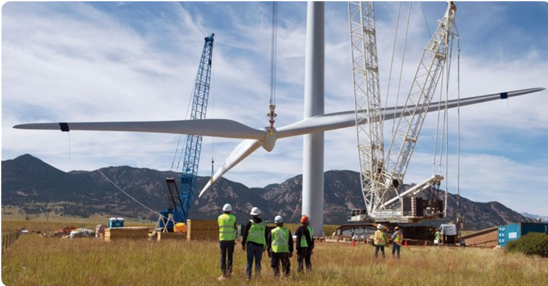
Lake Turkana Wind Power Project, Kenya.
