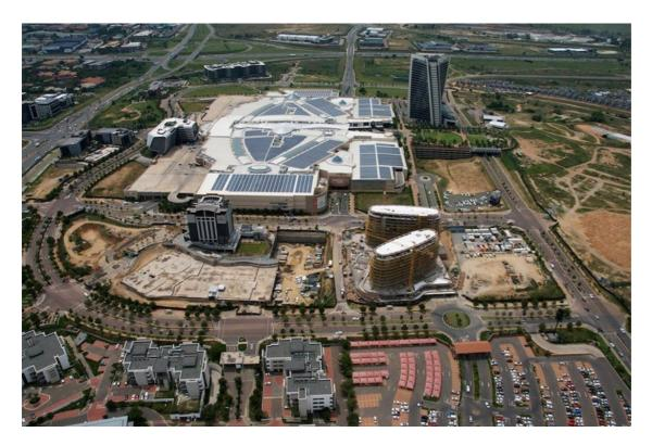
Despite the devastating impact of Covid-19 on the tourism and hospitality industry, construction of the new hotel has only been set back four months. In building this striking new property, some 4,095m³ concrete was used, 141tn of reinforcement, 9,865m² of post tensioning reinforcement of slabs, 15,919m² of brickwork, 2,400m² of glazing and 1,558m² of ventilated façade.
